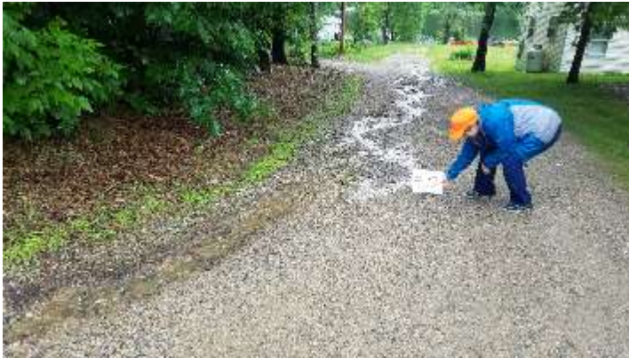
This high impact private road has sheet surface erosion, sheet erosion in a ditch, bare soil, and a steep slope directly to the lake
